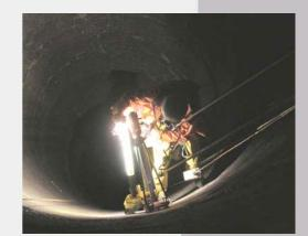
This underground station has 7 200m vertical penstocks through rock to feed the underground turbines. As part of the 30 year Half Life Refurbishment Project the penstocks required a concrete condition survey. They are lined with slipformed concrete and steel.
