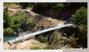
A 30-metre long, 1600mm wide, steel deck suspension bridge was chosen as the most cost-effective solution for getting small vehicles across the picturesque gorge. The cable anchors are RB25 drilled and grouted rock anchors. Access to both sides of the gorge was achieved by installing an aerial ropeway.
